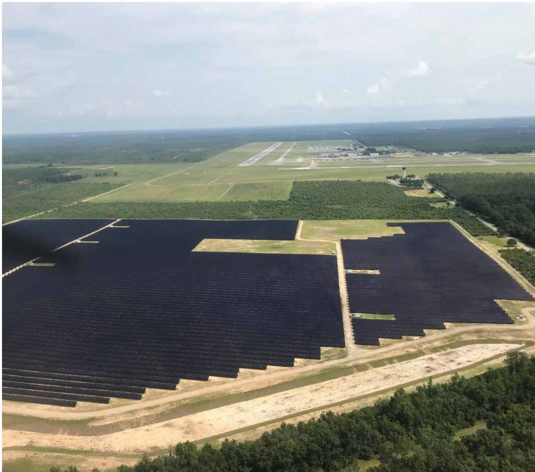
Figure 43. A 20 MW AC solar PV plant located at Tallahassee International Airport (pictured above) went into commercial operation December 13, 2017. The plant production supplies the City of Tallahassee Electric Utility and its first Community Solar program, which was soon fully subscribed. A second solar PV plant, rated at 42 MW AC , went into commercial operation at the airport on December 26, 2019, making the combined installation, at 62 MW AC , the world's largest airport-based solar facility [37]. (photo credit: J. Kearney, Nhu Energy)
